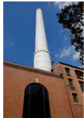
Incinerator chimney. Photograph: Jon W
