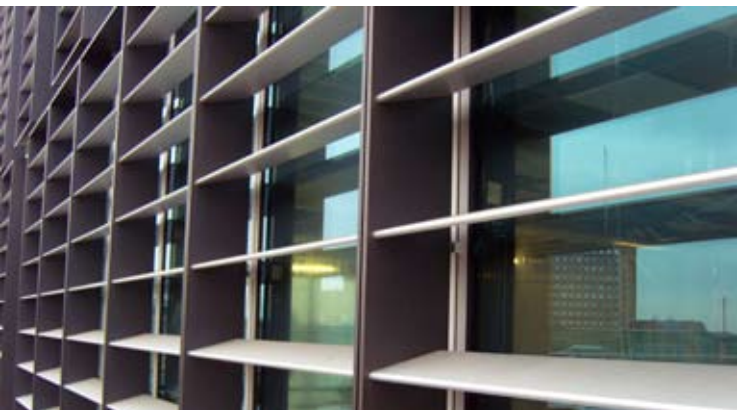
Solar shading on the new offices of East Thames Group
