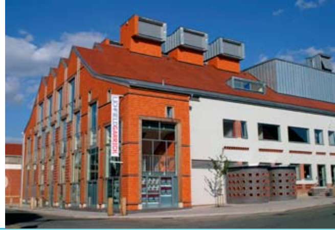
Lichfield Garrick: A fully naturally ventilated arts space
