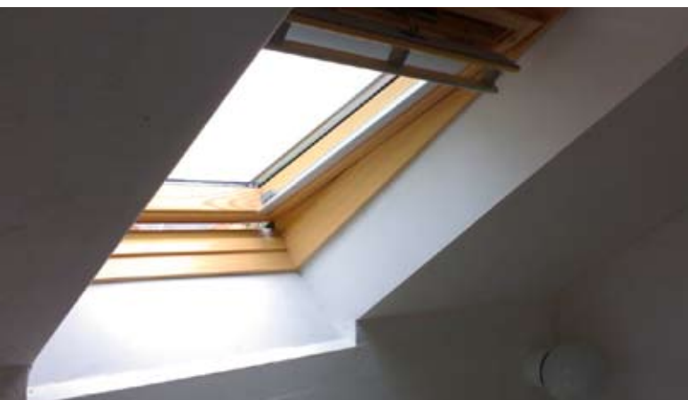
Velux roof light Photograph: Robert Brook
