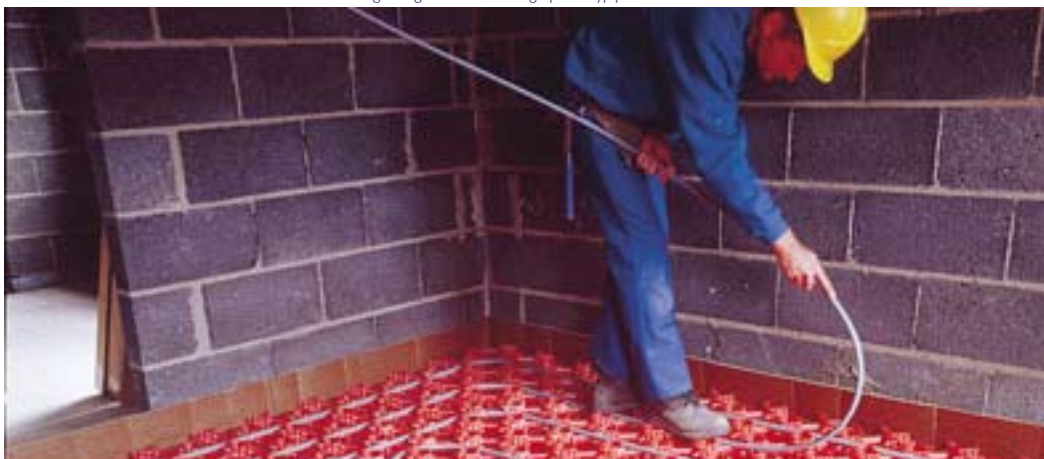
Underfloor heating being installed. Photograph: Polypipe
