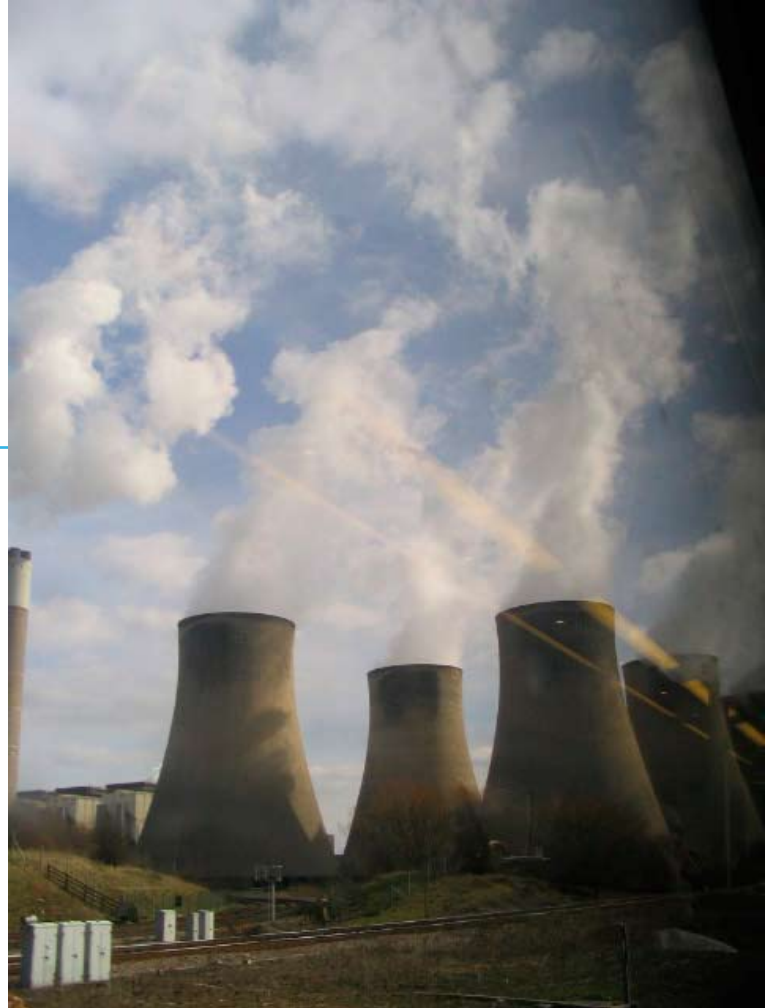
Drax coal-fired power station, North Yorkshire. Photograph: La Petite Claudine
