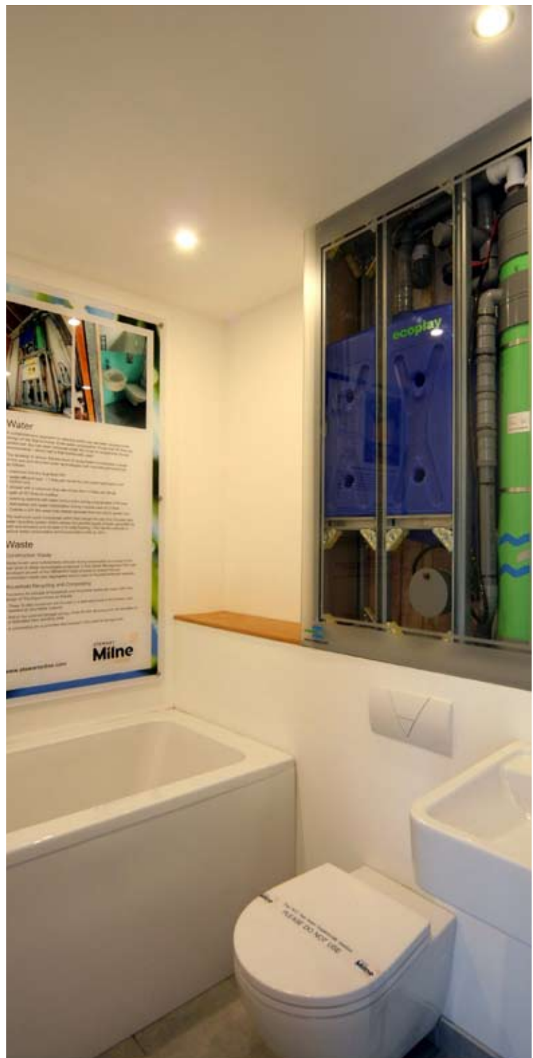
Ecoplay grey water recycling system Photograph: PRP Architects
