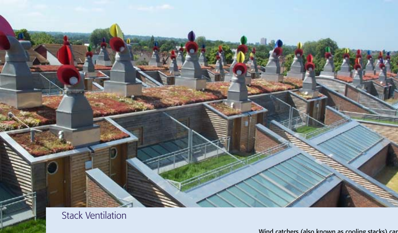
Wind Catchers at BedZed Zero Emissions Development
